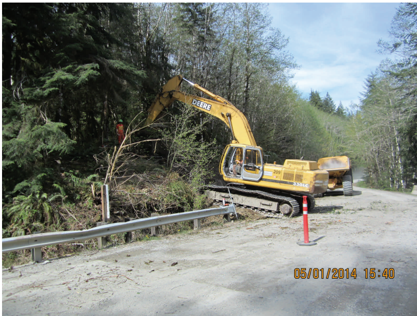
Above: Excavation at the 588+50 Bridge begins
