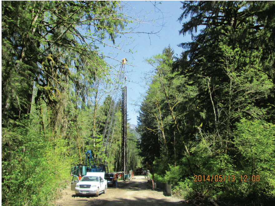
Above: Pile Driving at the Timber Bridge
