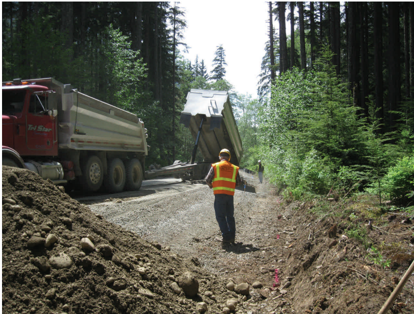
Above: Placing roadway fill near Middle Fork trailhead.
