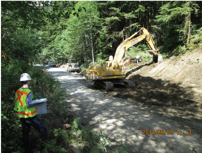
Above: Excavation to widen the road near the 588+50 bridge.
