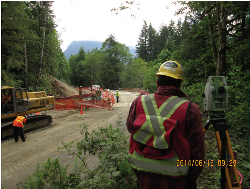
Above: Surveying pile locations at the 588+50 bridge.
