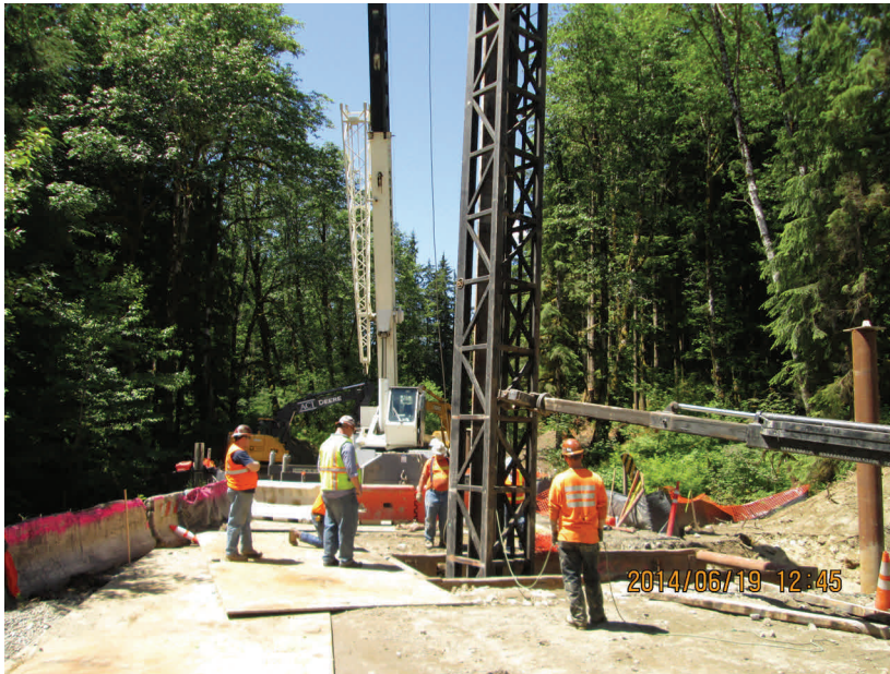
Above: Pile driving at the 588+50 bridge.
