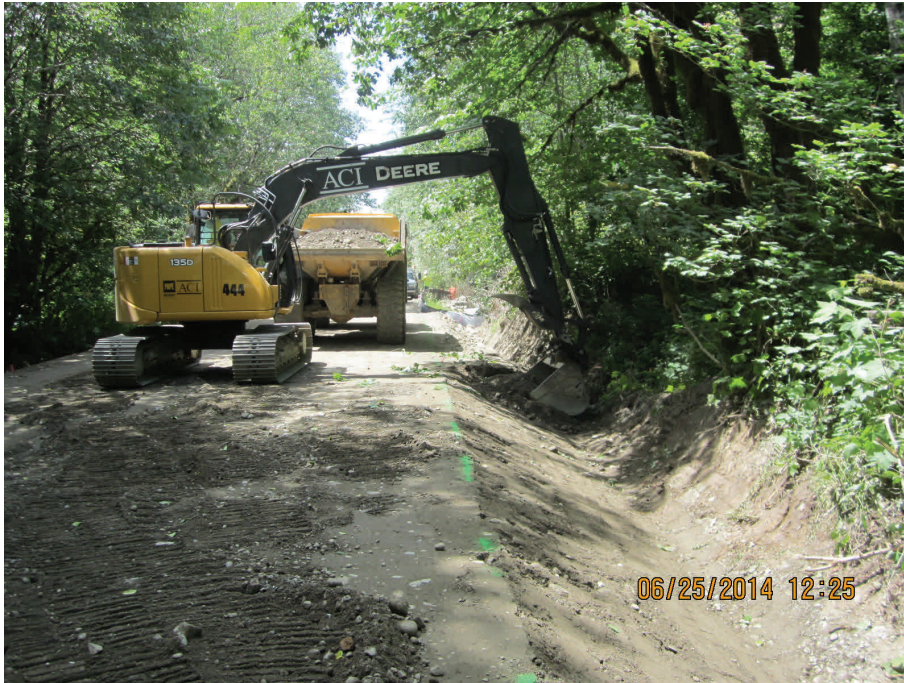
Above: Finishing roadway slopes.
