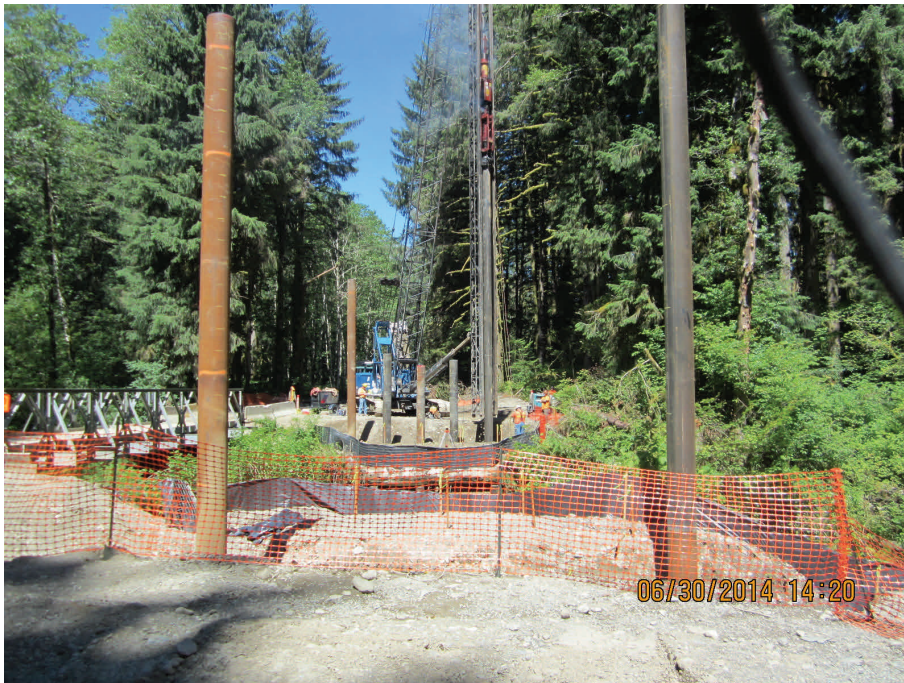
Above: Completing pile driving at the 471+85 bridge over Big Blowout Creek.
