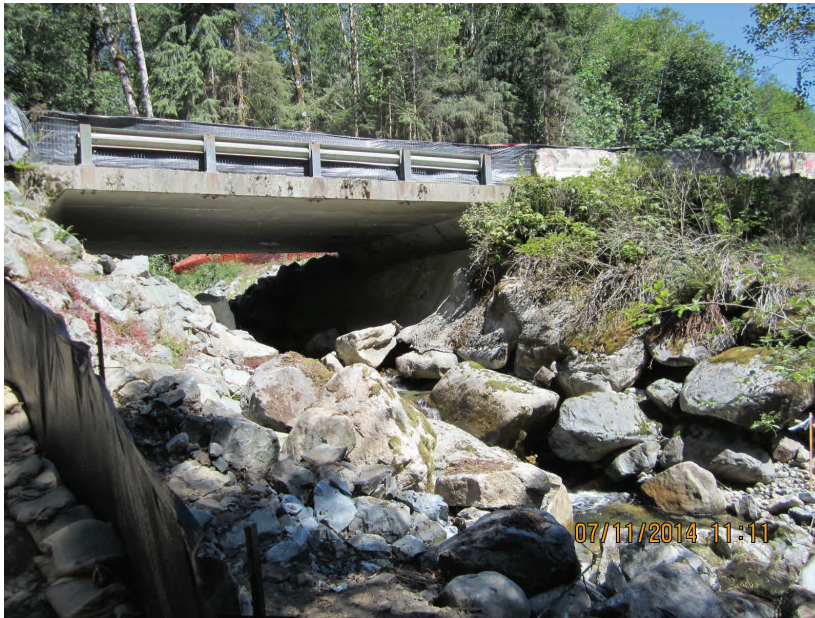
Above: Existing 588+50 bridge.
