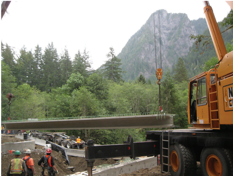
Above: Setting girders at the 588+50 bridge.
