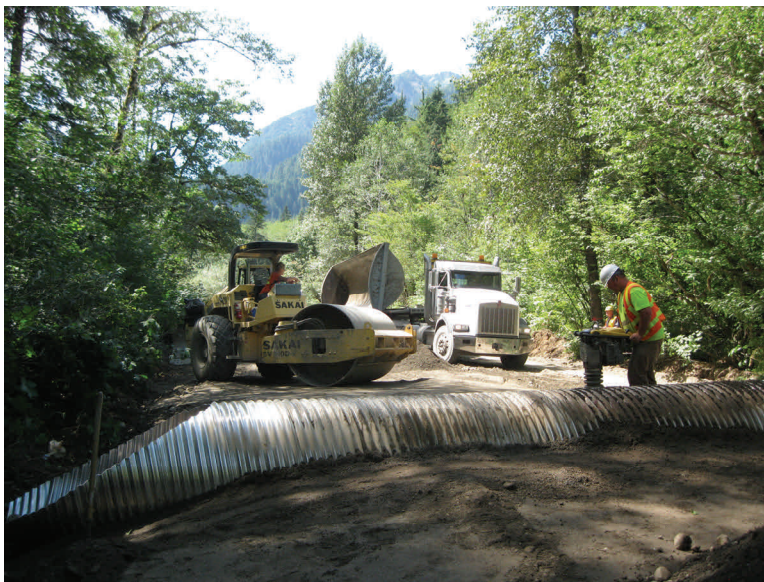
Above: Culvert installation.
