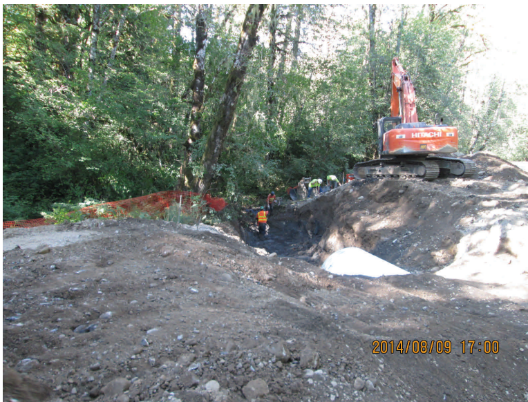
Above: Constructing an aquatic organism passage culvert pipe.
