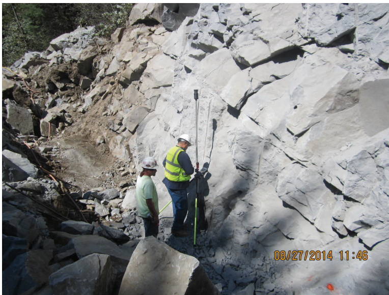
Above: Checking the finished rock blasting at the CCC trail connection.
