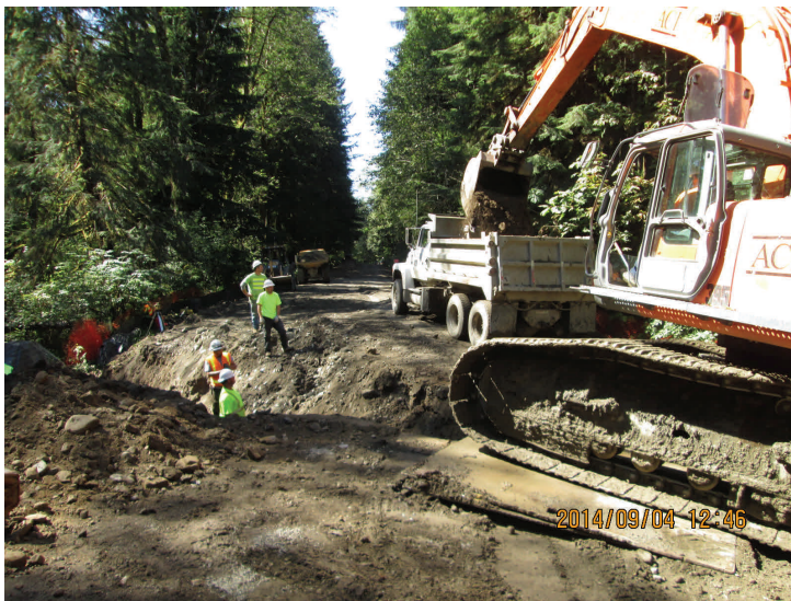
Above: Excavating for a large culvert pipe.
