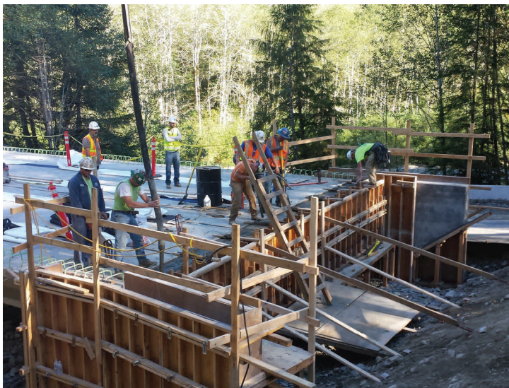
Above: Placing concrete in the end wall on the 588+50 bridge.
