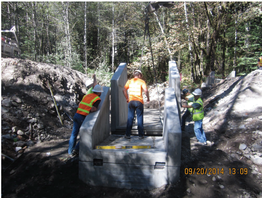
Above: Installing a precast concrete box culvert.
