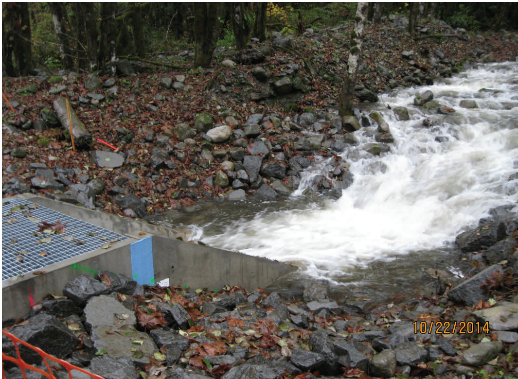
Above: Stream flowing through a completed box culvert.
