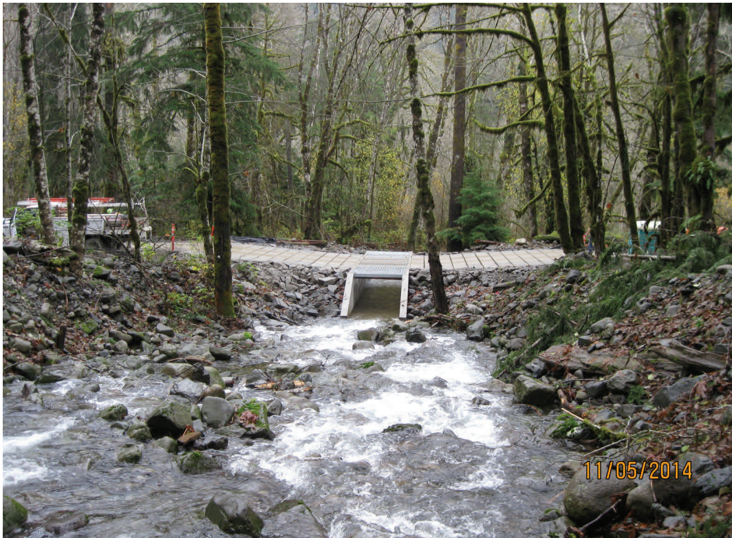
Above: Completed low water crossing.
