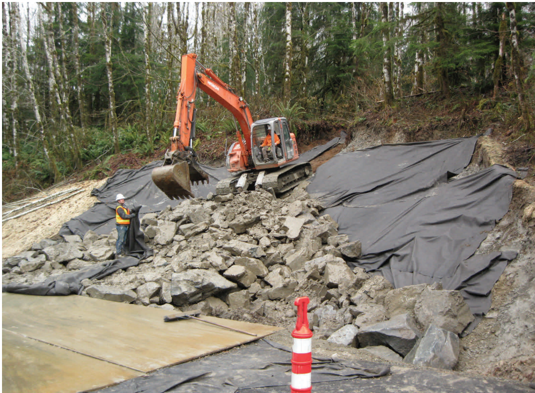
Above: Constructing a rock stabilized slope.
