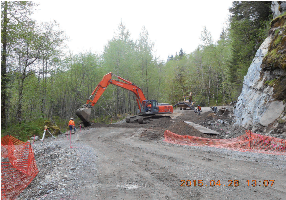
Above: Working on the slide near the CCC trail.
