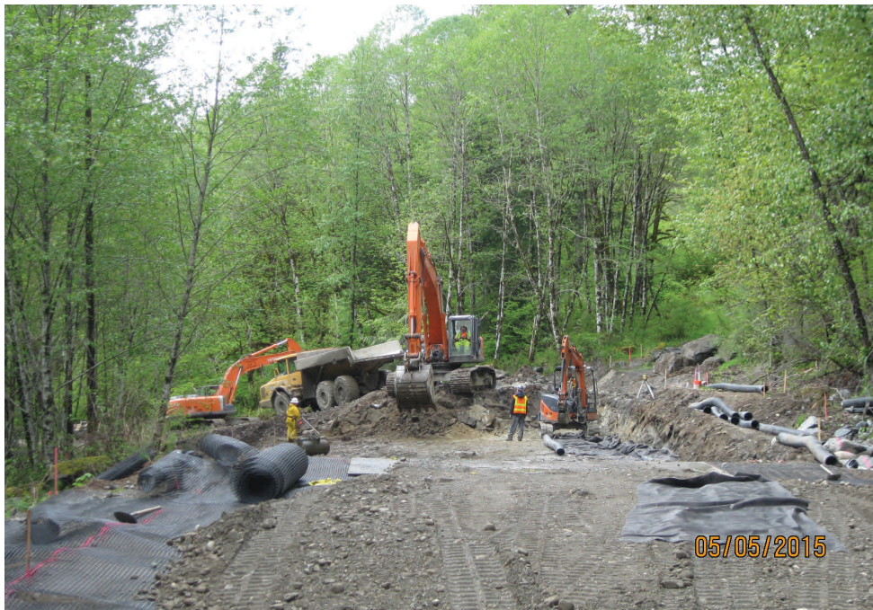
Above: Constructing a reinforced roadway over the slide near the CCC trail.
