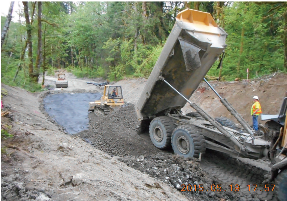
Above: Constructing the roadway over soft soils.
