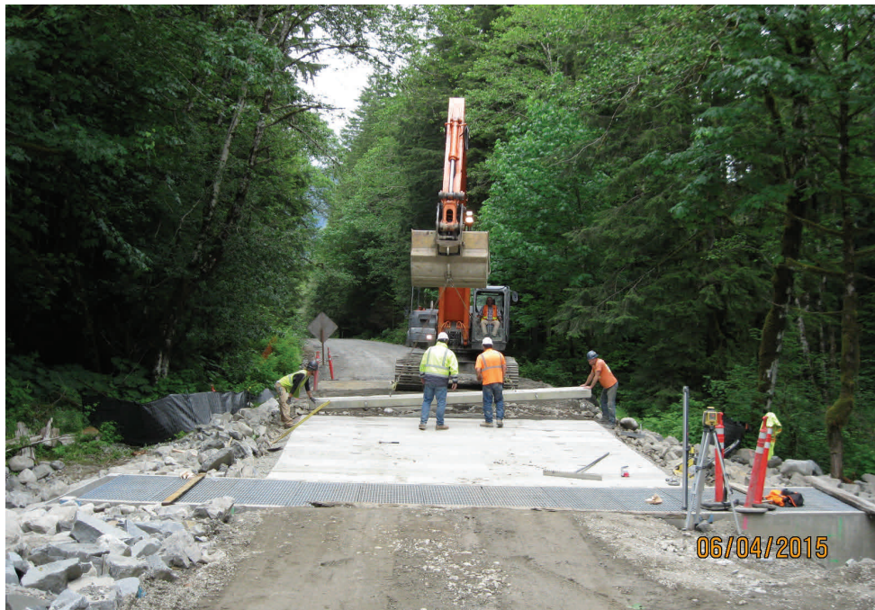
Above: Strengthening and repairing the damaged low water crossings.
