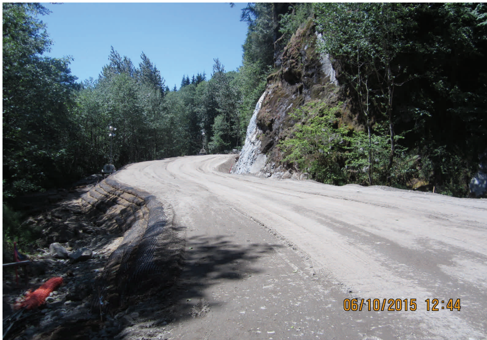
Above: Reinforced roadway crossing the slide area near the CCC trail.
