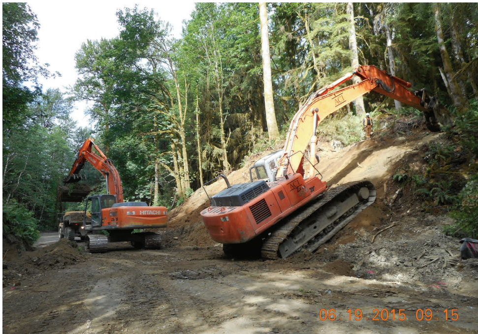
Above: Excavating new roadway cut slopes and ditches.
