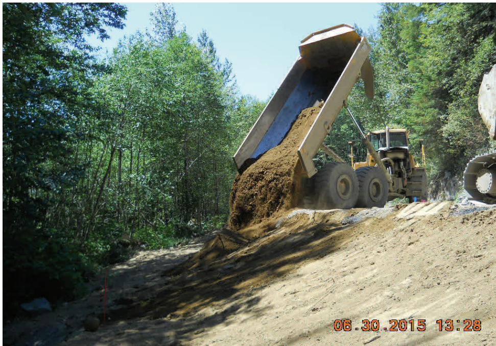
Above: Placing topsoil on the finished roadway slope.
