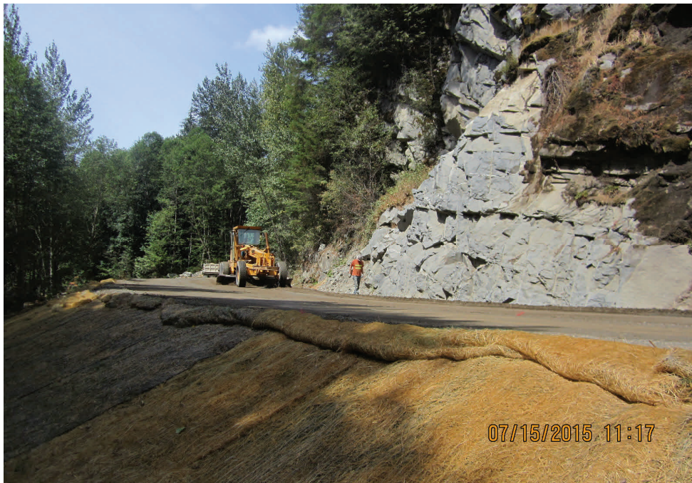
Above: Finishing the roadway near the CCC trail.
