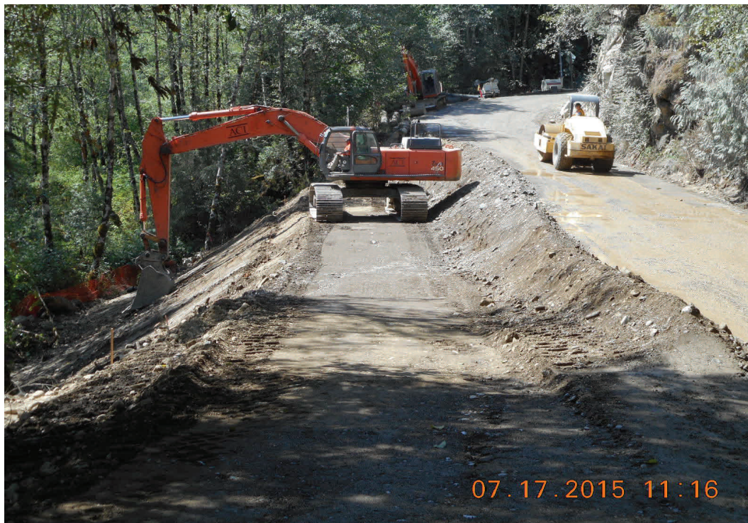
Above: Placing fill to widen the roadway.
