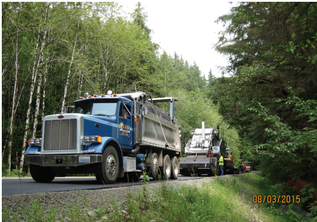
Above: Paving was completed this week between the two new bridges.
