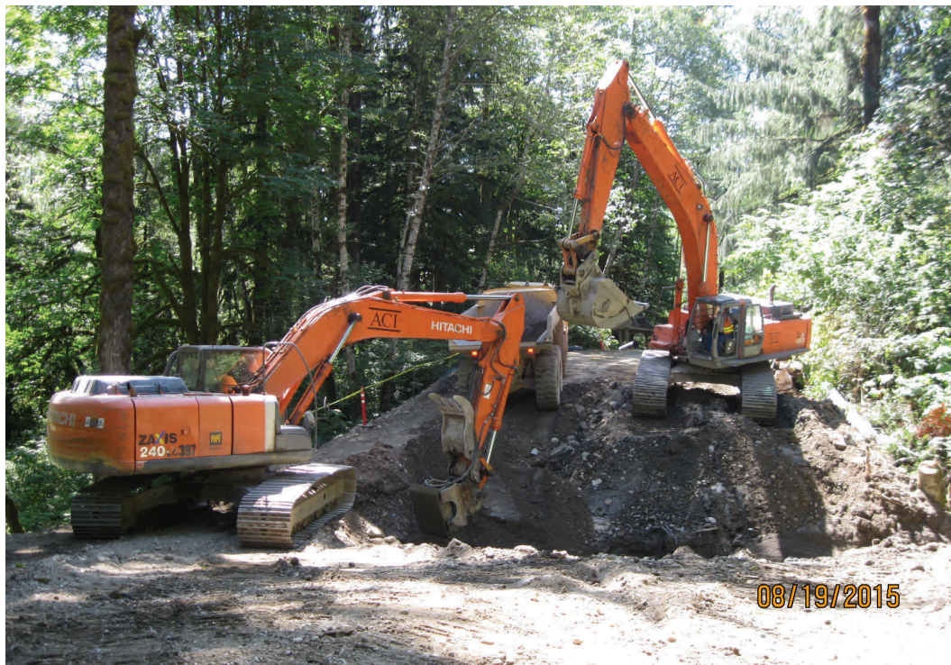
Above: Excavating for a culvert pipe near Bessemer Road.
