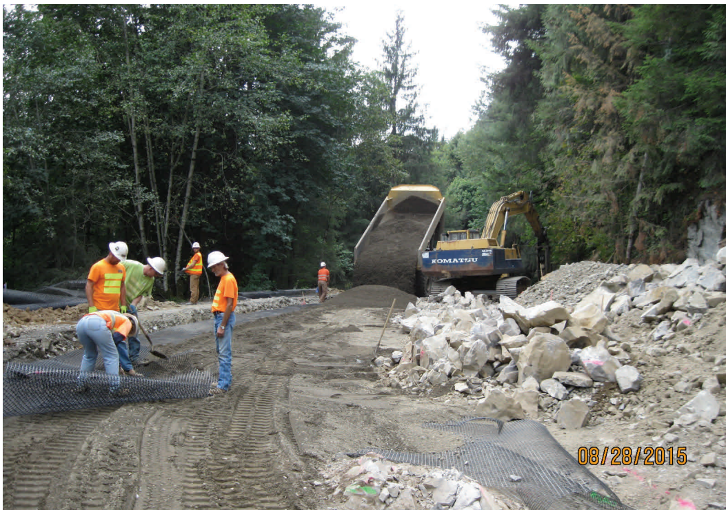
Above: Constructing reinforced roadway.
