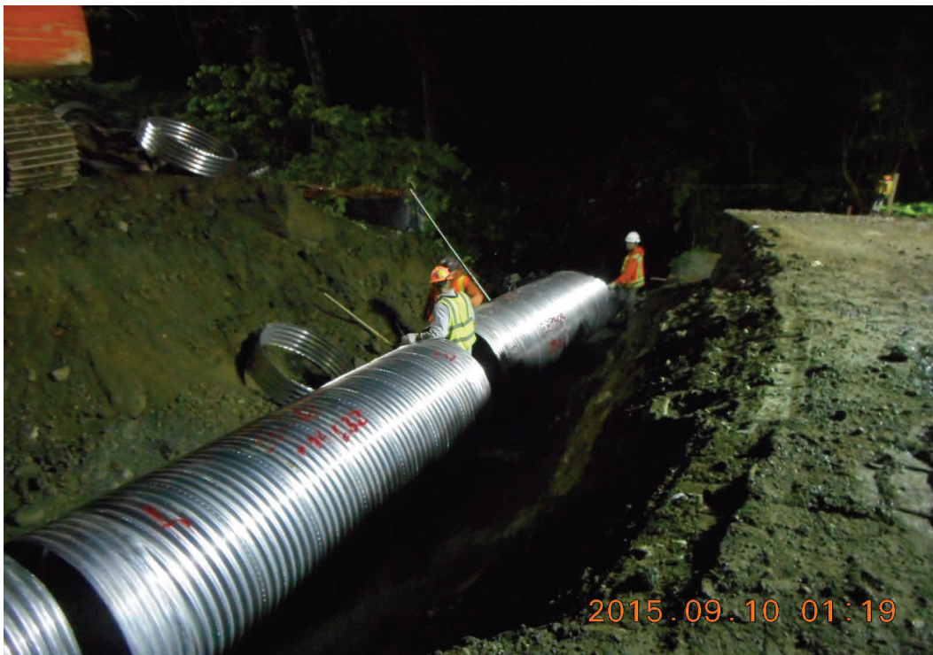
Above: Culvert installation.
