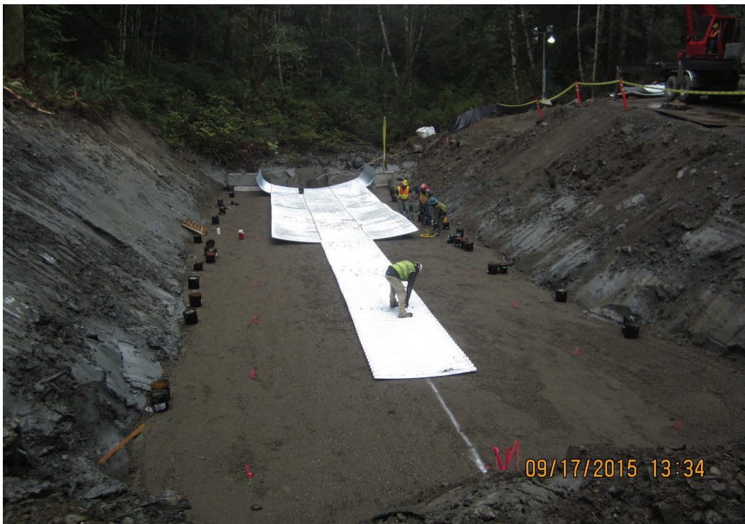
Above: Culvert assembly.
