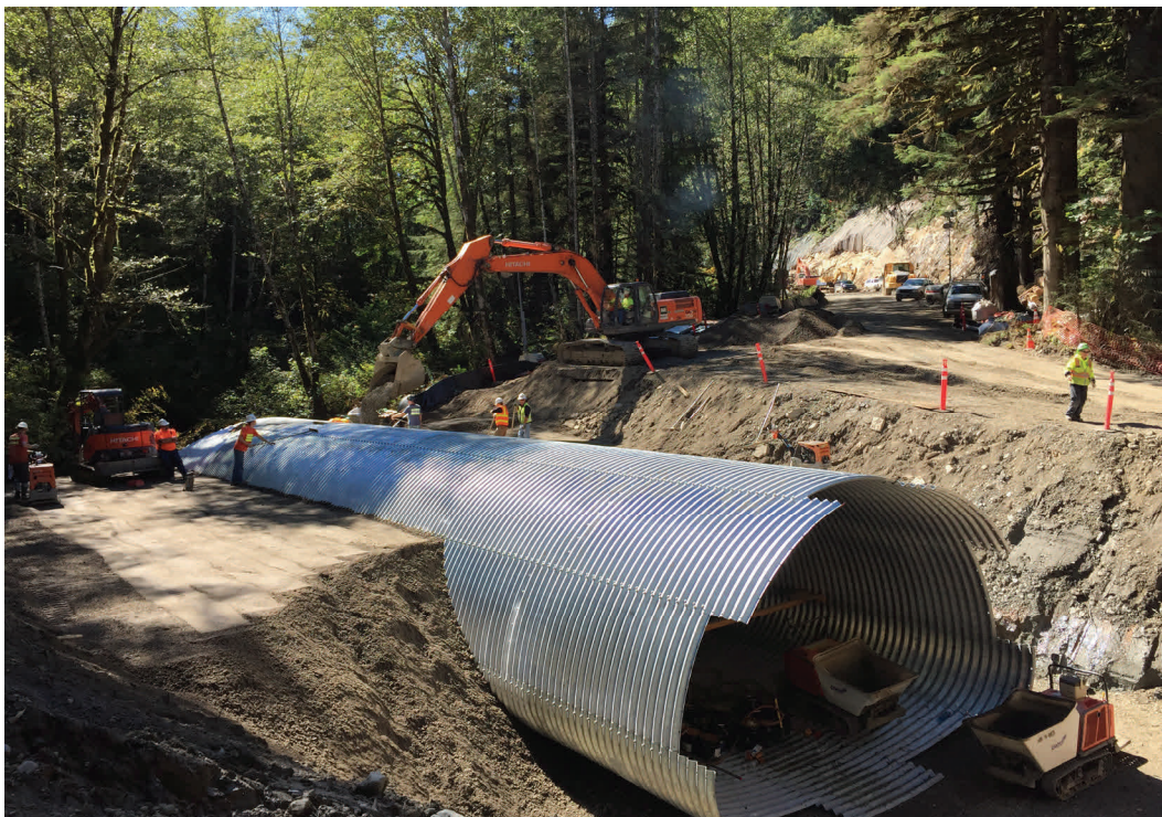
Above: Backfilling the large culvert..
