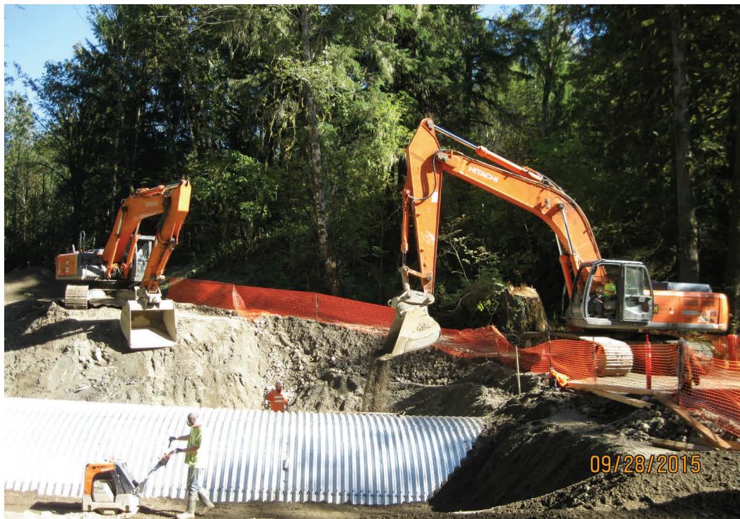
Above: Backfilling the final stage of the large culvert.
