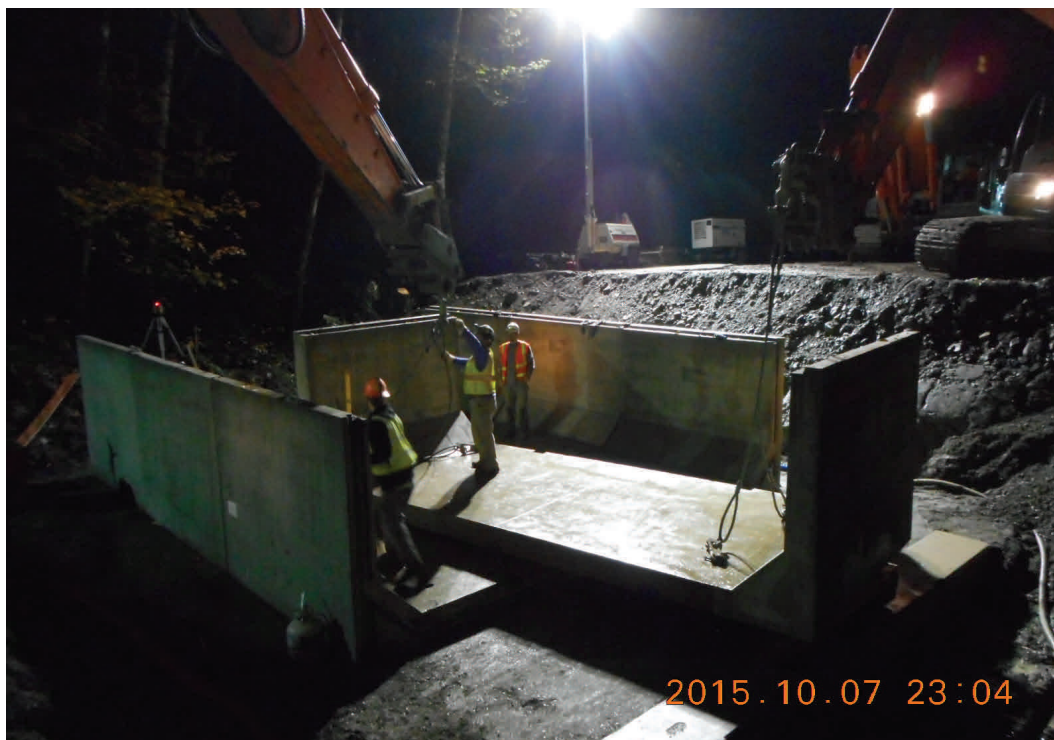
Above: Setting precast concrete box culvert sections.
