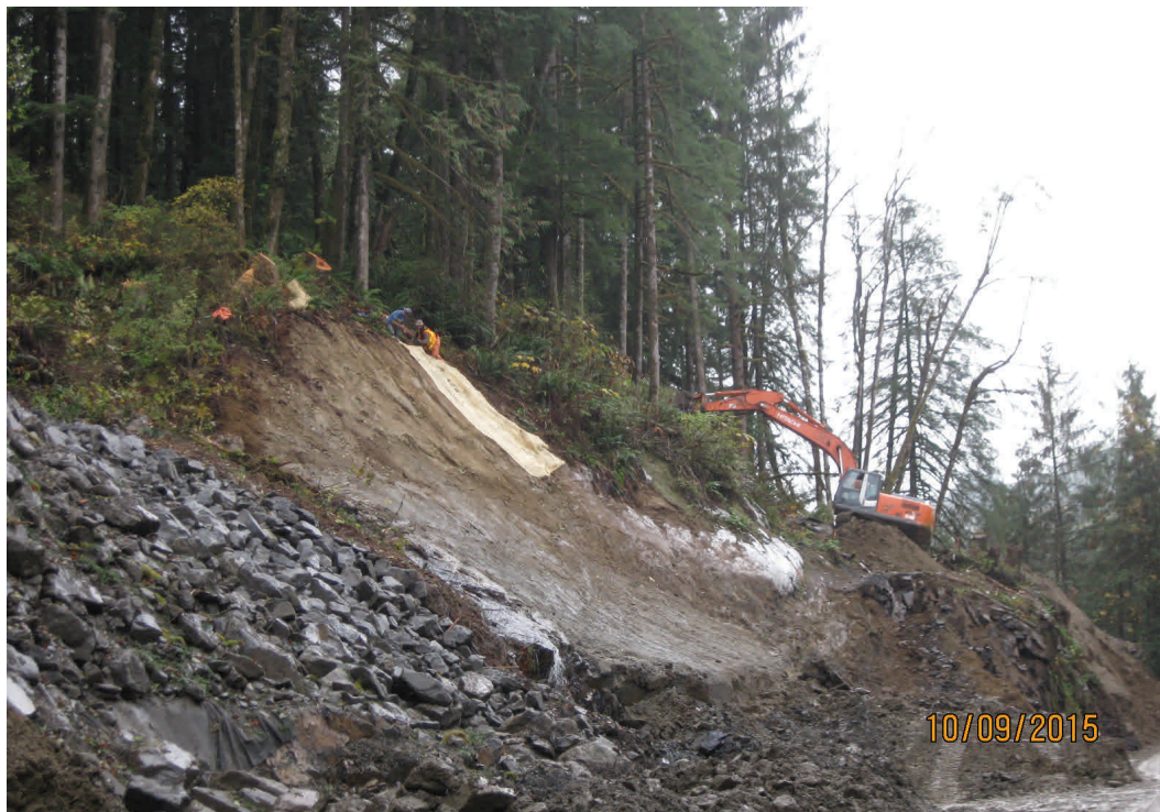
Above: Cut slope repair.
