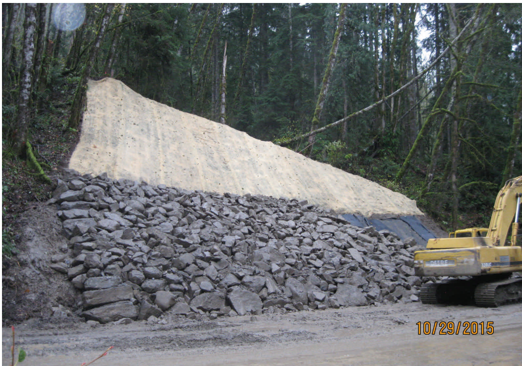
Above: Constructing a rock supported slope.
