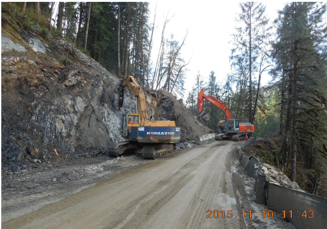
Above: Rock excavation.
