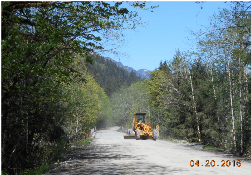
Above: Blading the roadway.
