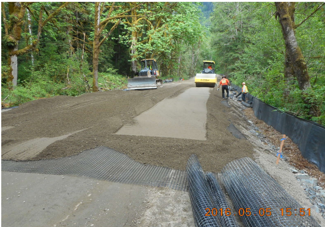
Above: Constructing reinforced roadway near Valley Camp.
