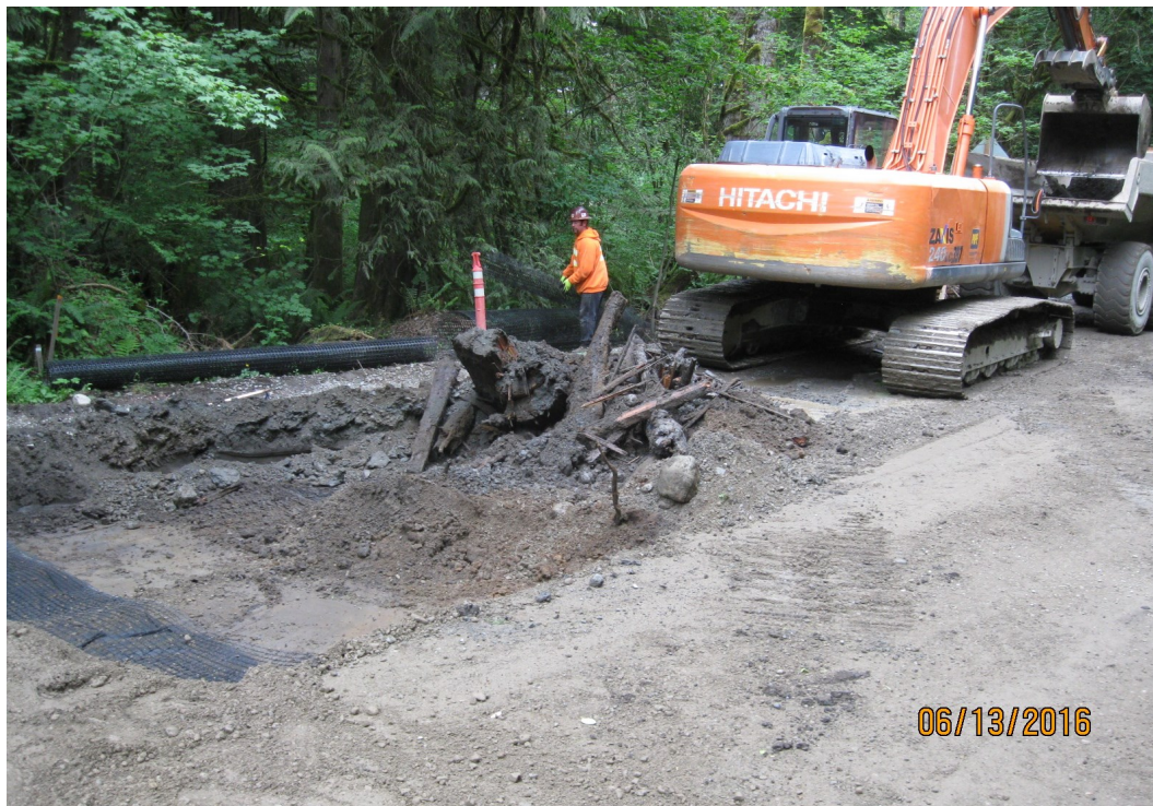
Above: Excavating unsuitable roadway fill near Valley Camp.
