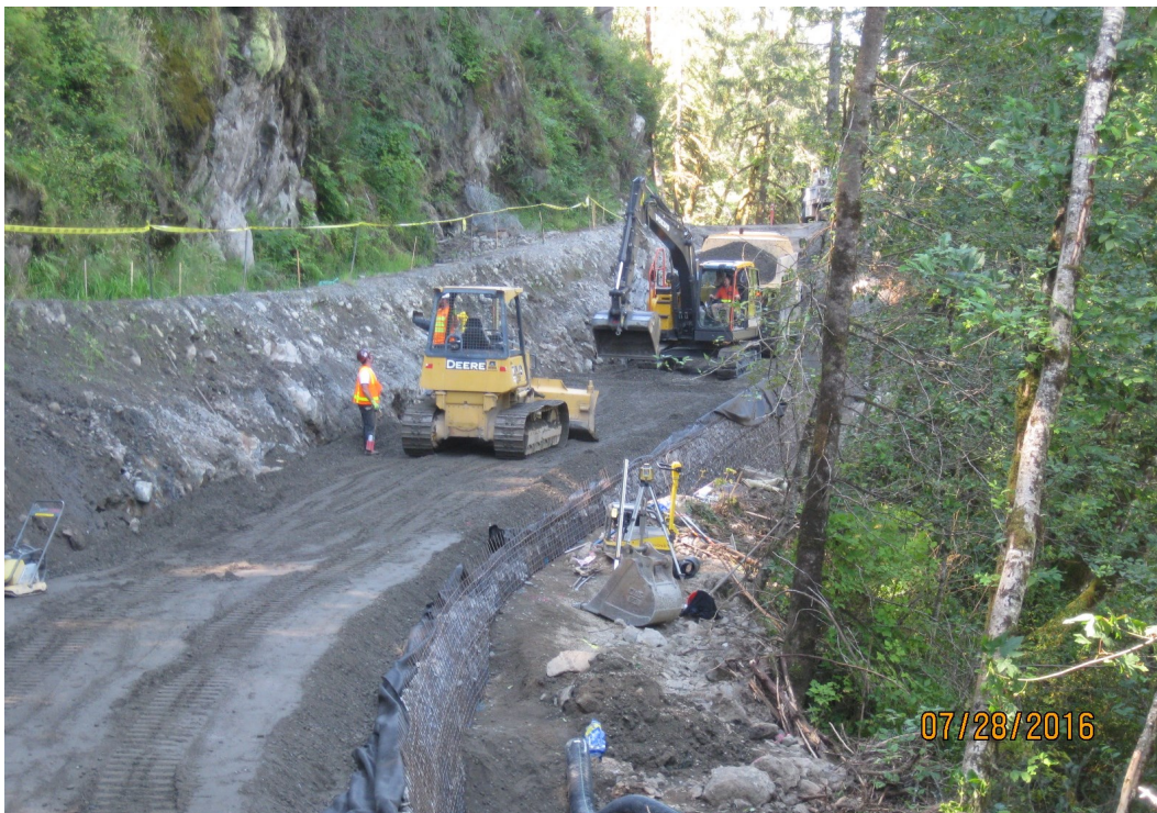
Above: Retaining wall construction.
