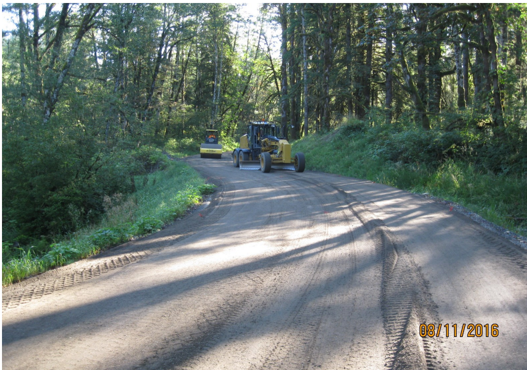
Above: Grading roadway surfacing near Oxbow to prepare for paving.
