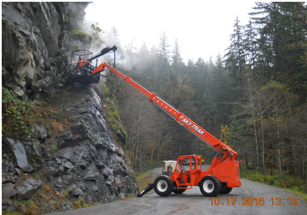
Above: Drilling for rock dowel installation near the CCC Trail.
