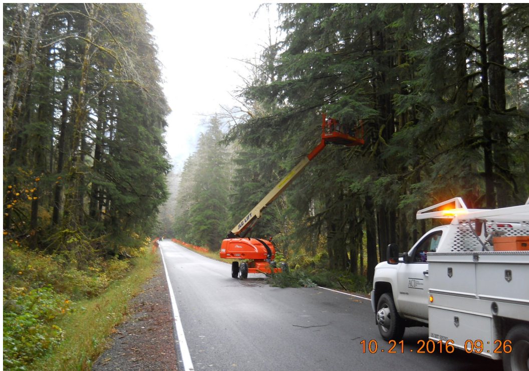
Above: Trimming trees above the completed roadway.
