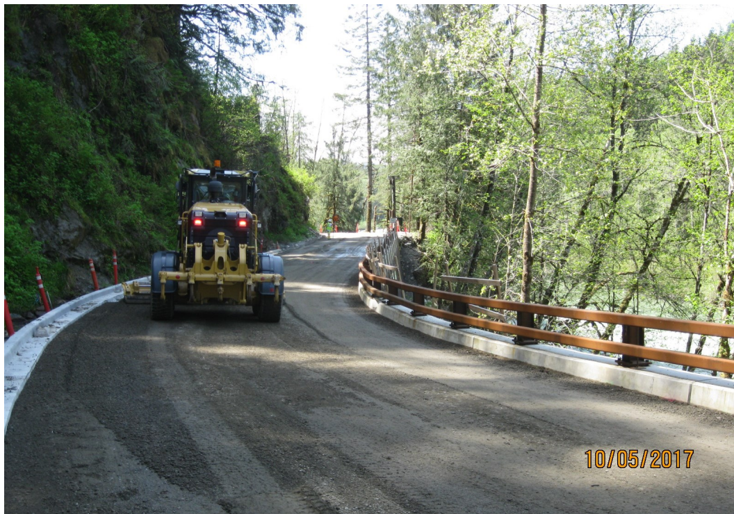
Above: Grading the road for paving near Champion Beach.
