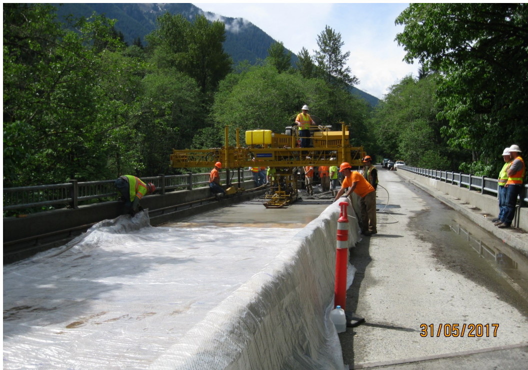
Above: Lake Dorothy Bridge concrete overlay.
