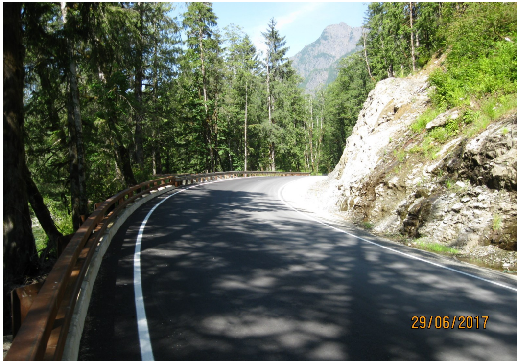
Above: Completed roadway near Champion Beach.
