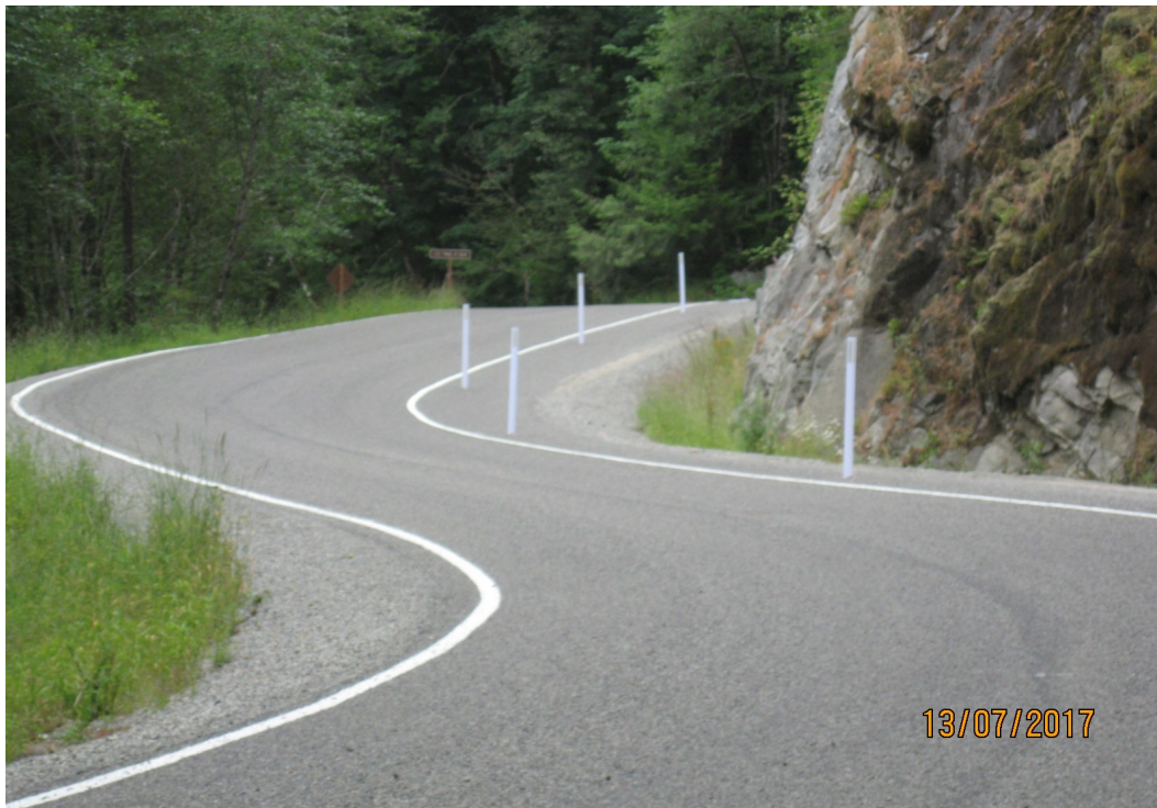
Above: Completed roadway near the CCC trail.
